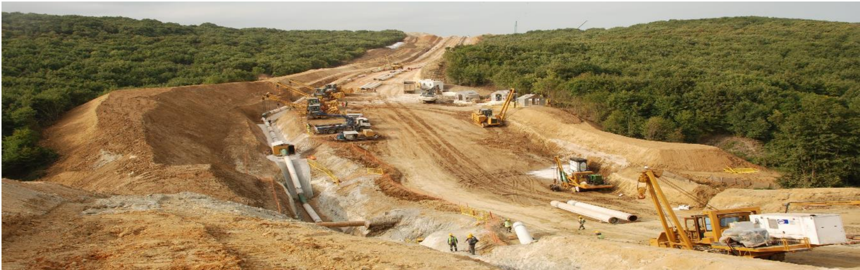
Figure 7 Onshore pipe-laying process in Kiyikoy (Schematic and Actual)
