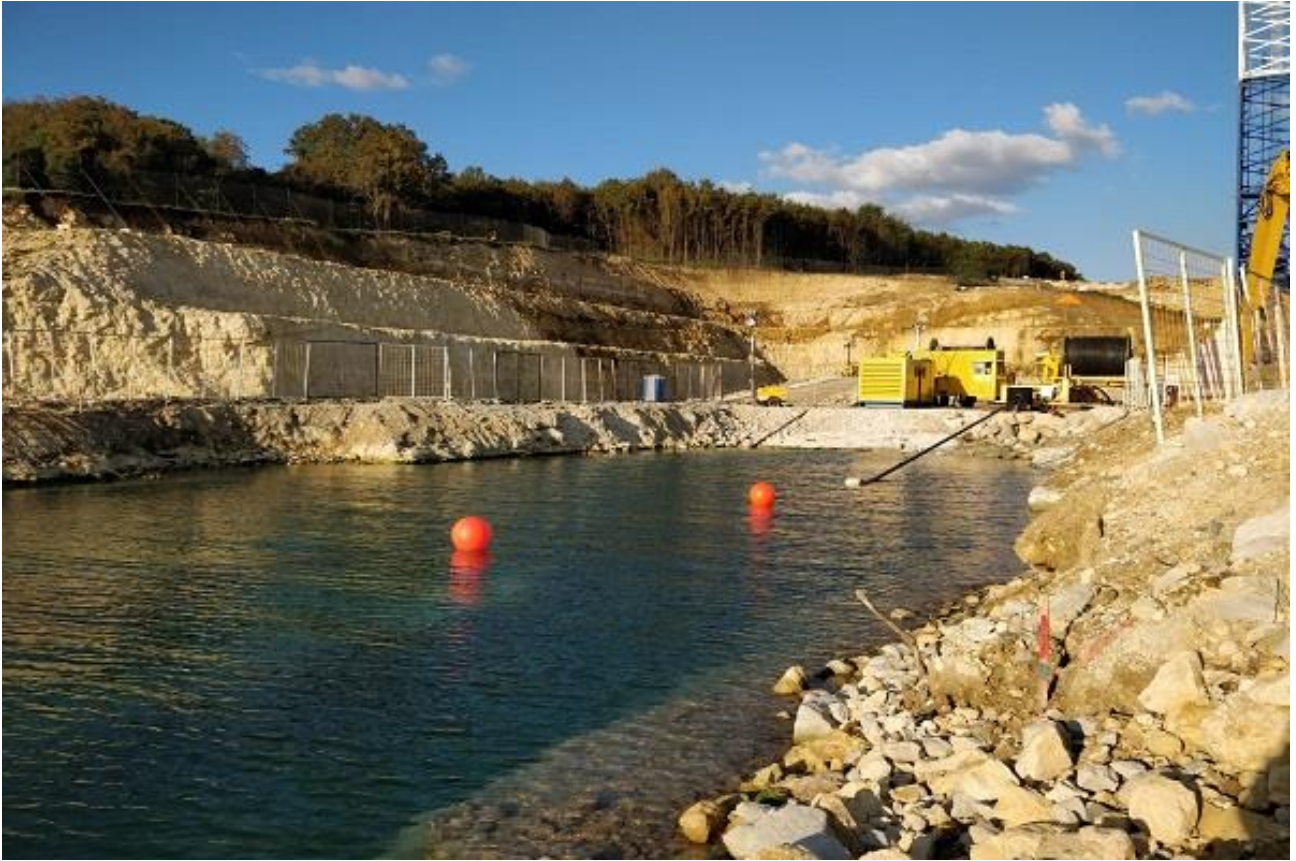
Figure 11 Shore pull operation in the nearshore
