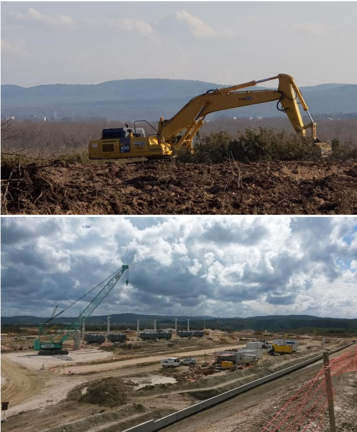
Figure 5 Land clearance and building of the Receiving Terminal
