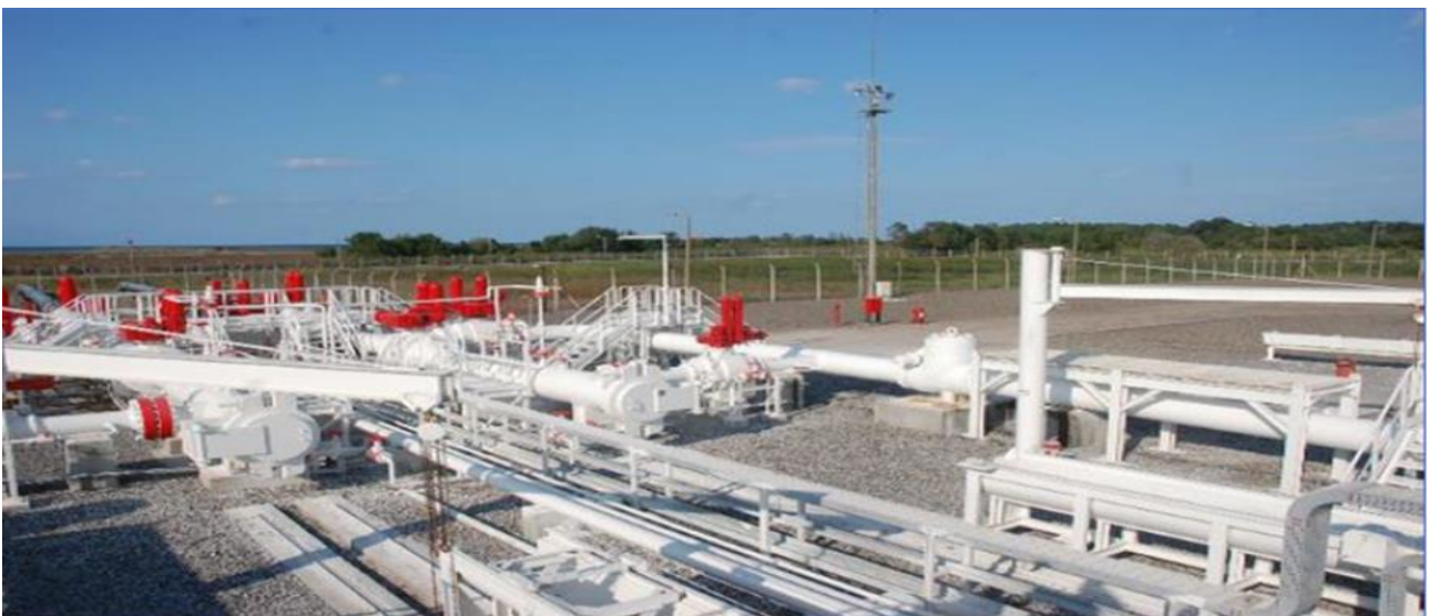
Figure 6 Example of a Receiving Terminal
