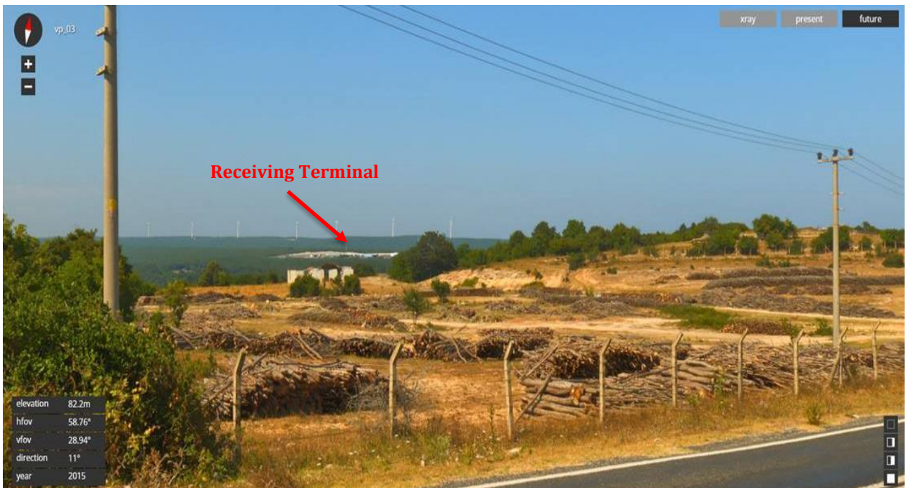
Figure 22 Visual of Receiving Terminal - Kiyikoy - Vize Road
