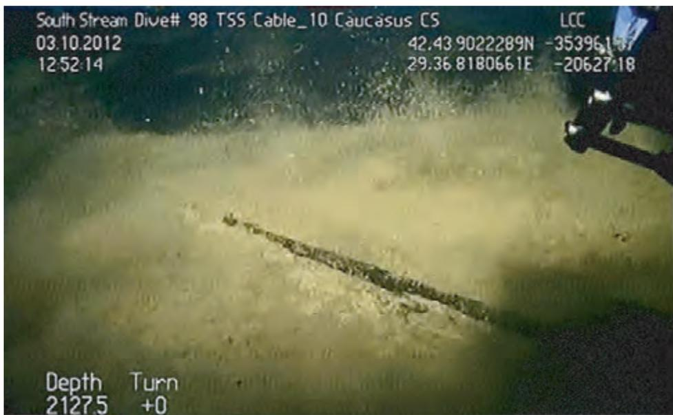
Figure 87. Still images derived from ROV video of a telephone cable exposed at the seabed.
