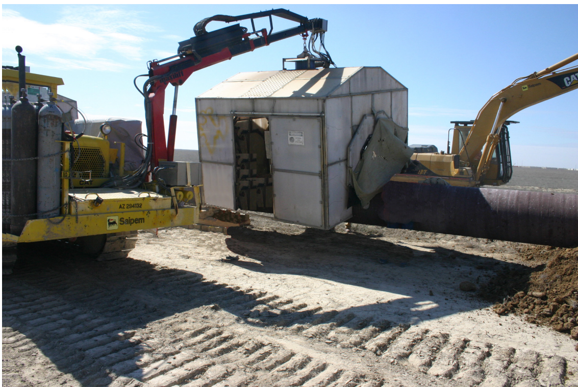
Figure 5.15 Pipe Welding Shelter
