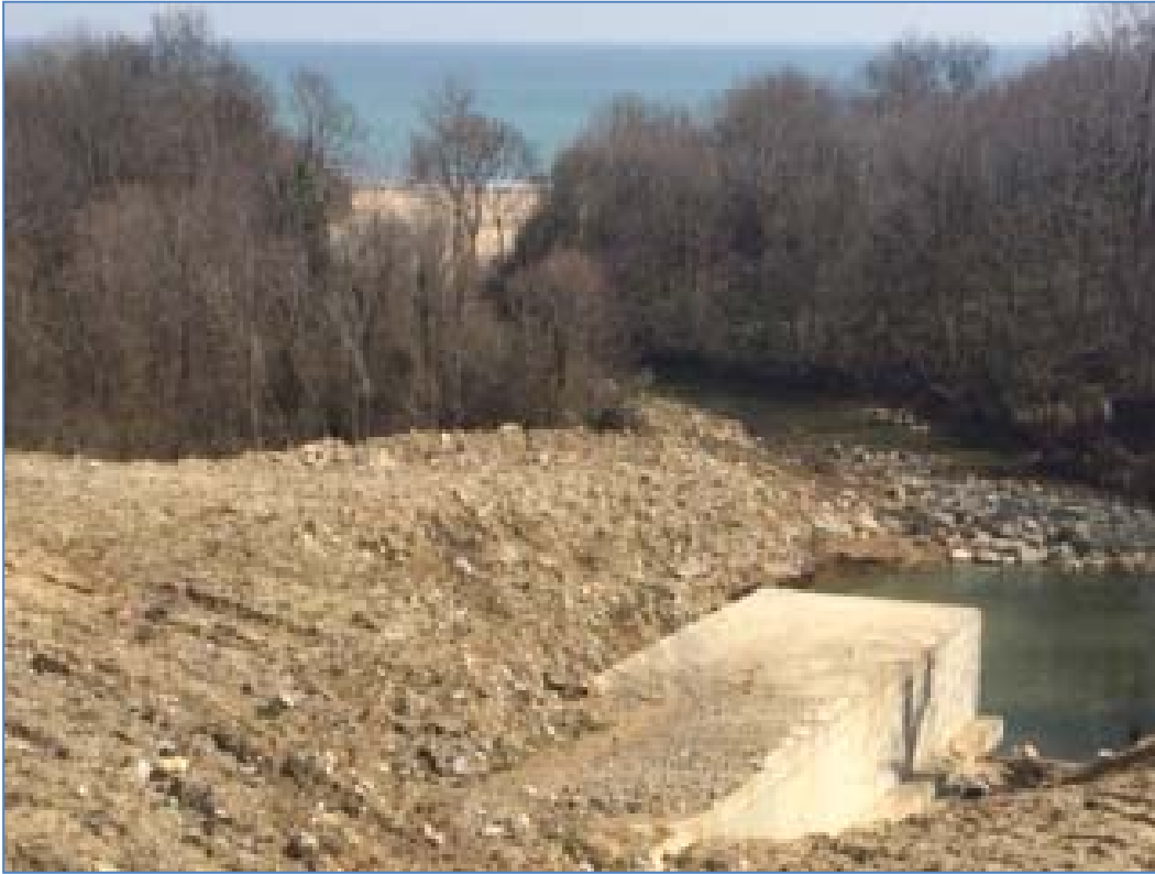
Figure 6.73: The structure of the culvert built under the soil in the Sazlıdere stream bed near to the sea shore (It is built to provide access to İSKİ's water pipeline connecting to Pabuçdere Dam Lake and covers the stream bed transversely as well as lying in parallel to the sea shore. The image is taken to the seaside (41°39'18.77"N/ 28° 5'4.34"E).).
