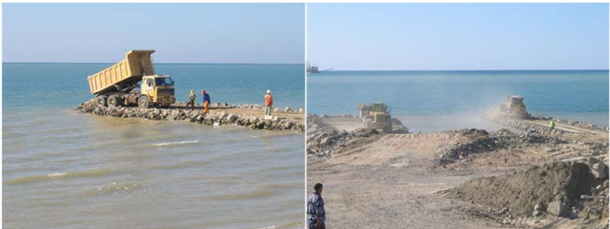
Figure 1.16: Causeway construction: dump truck (left) supported by shovel and bulldozer (right)
