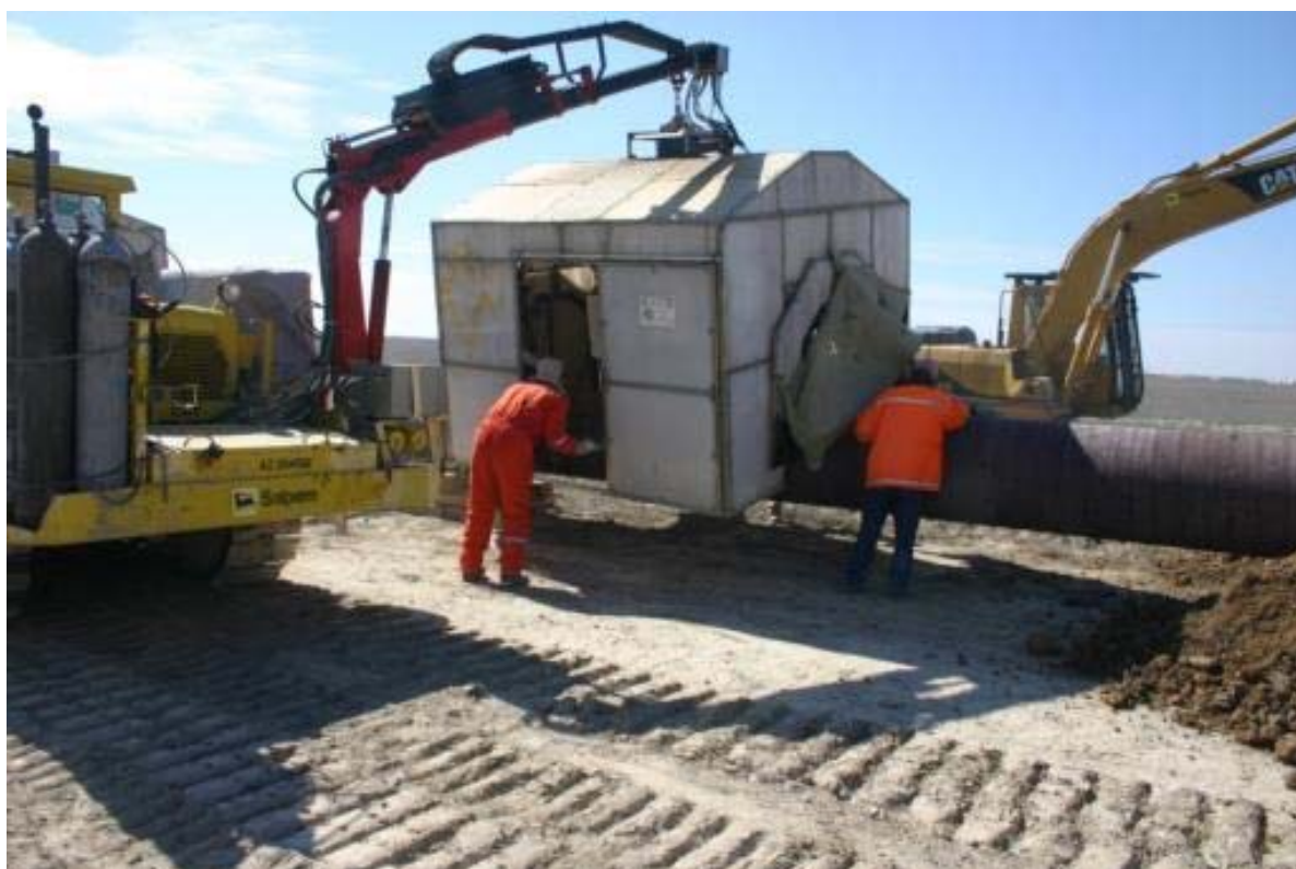
Figure 1.26: Pipe Welding Shelter
