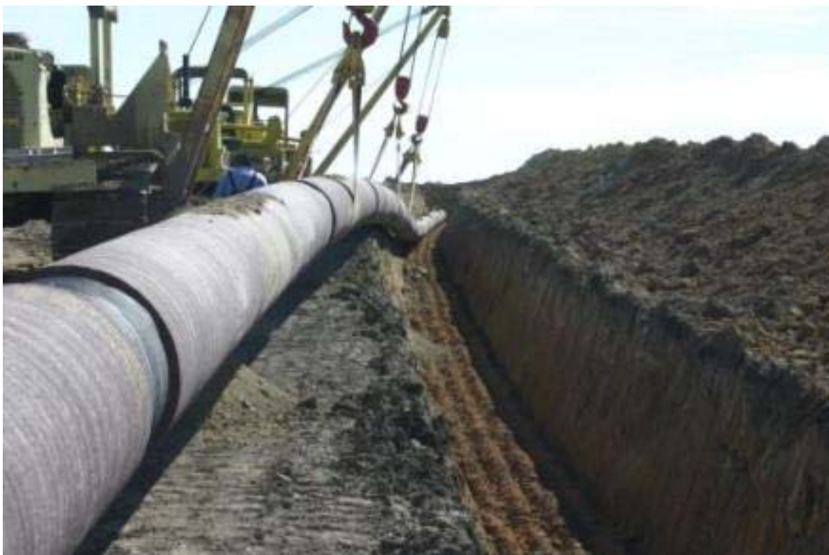
Figure 1.30: Pipe lowering into the Trench
